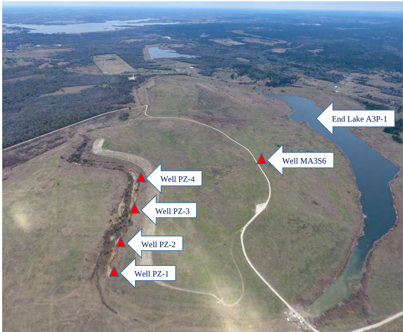
Figure 2 – Aerial view of Seep 9A Project (as of 05/26/21)
