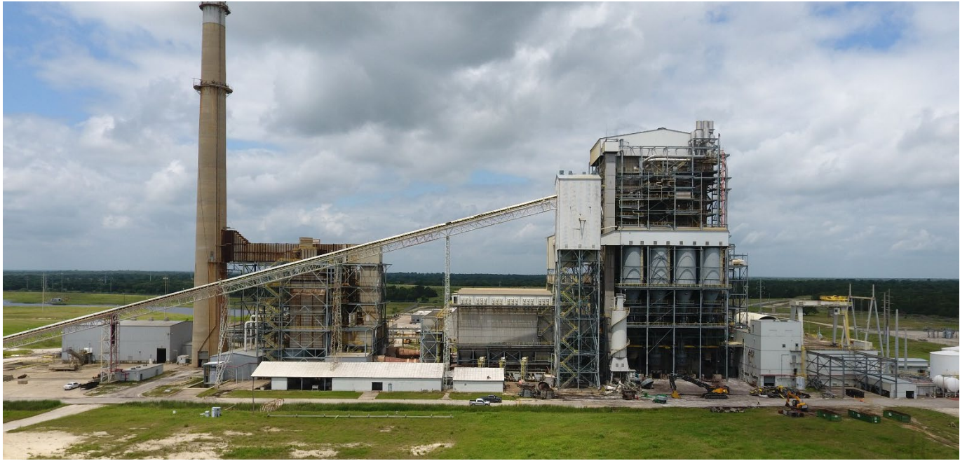
Gibbons Creek Steam Electric Station – May 2021
