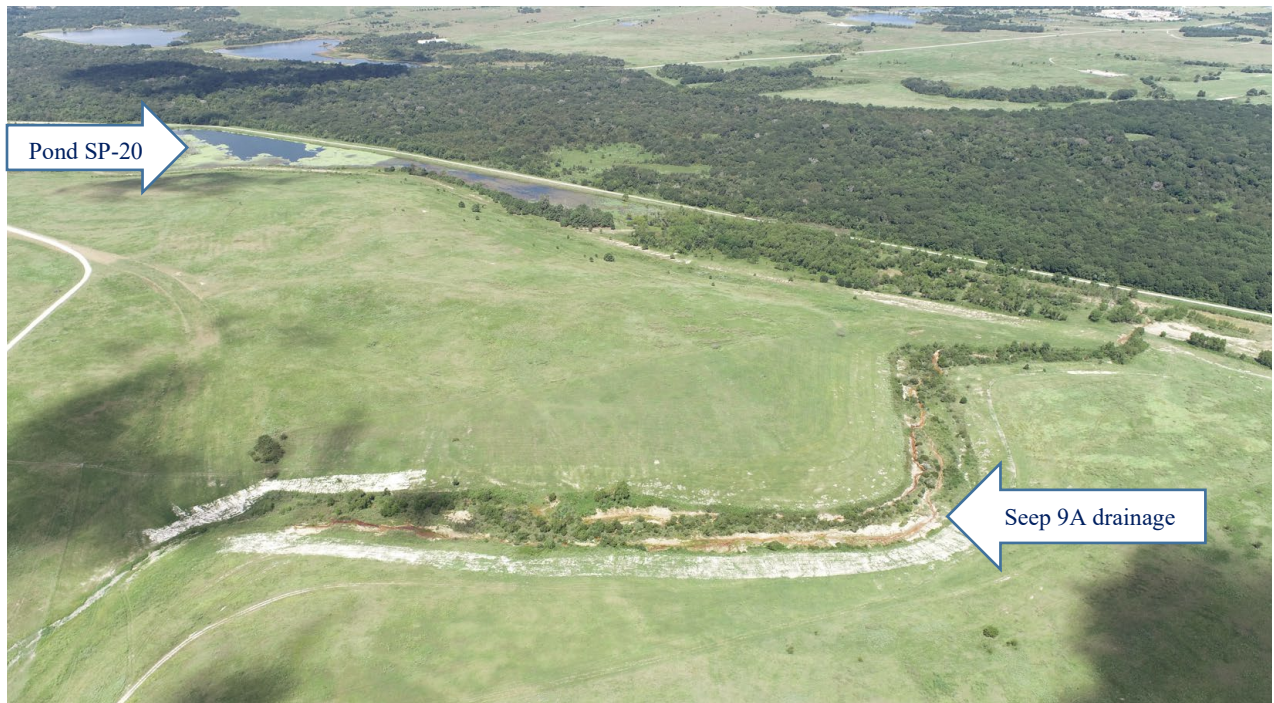
Figure 2 – Aerial view of Seep 9A Project (as of 08/24/21) (View northwest)
