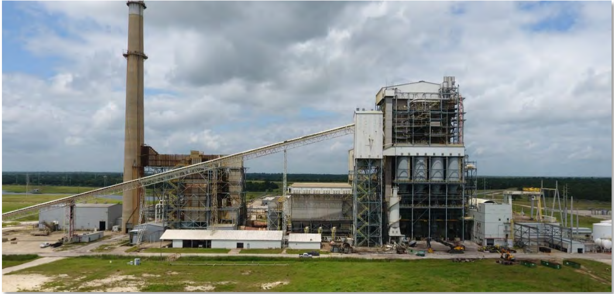
Gibbons Creek Steam Electric Station – May 2021
