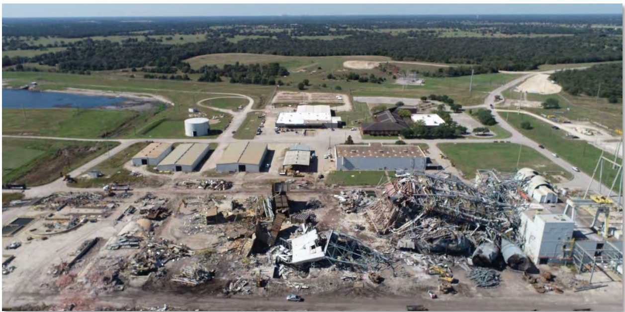
Gibbons Creek Steam Electric Station – November 2021
