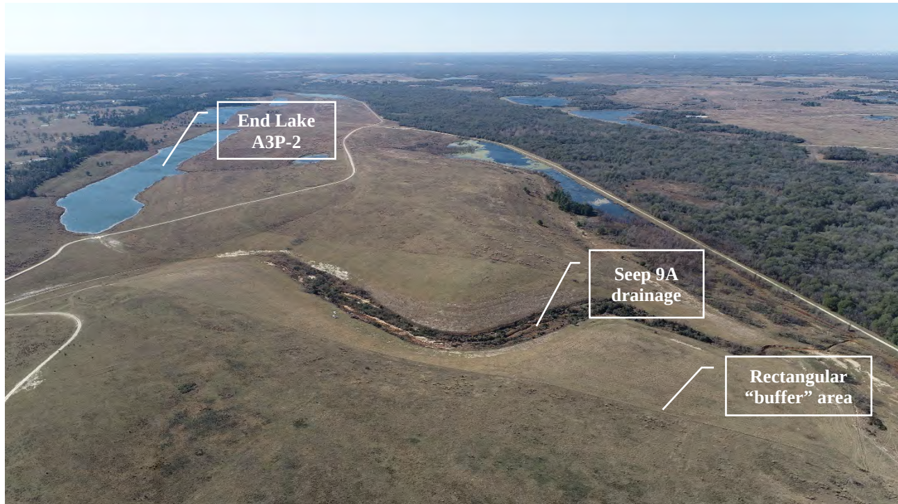
Figure 4 – Seep 9A Area showing rectangular bonding boundary (01/4/22)
