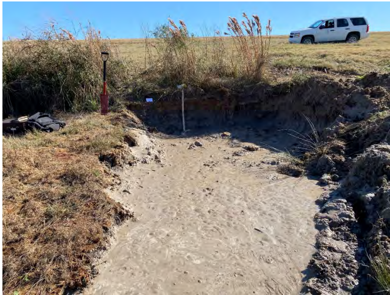
Figure 5 – Seep 9A drainage – Soil profile at toe of side-slope (view east, 01/4/22)
