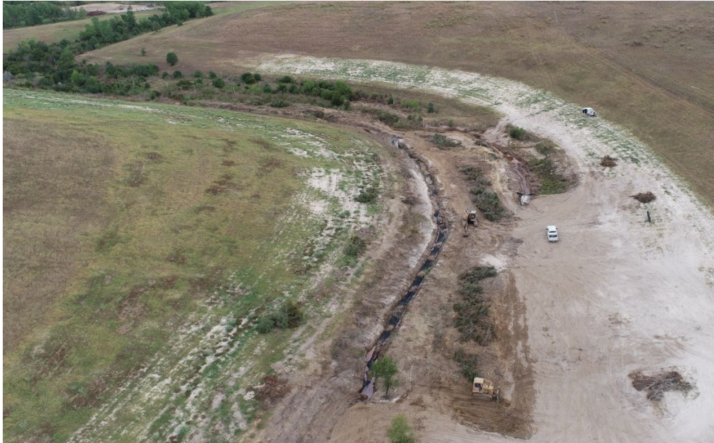
Fig. 3 – Status of Seep 9A mitigation work as of August 18, 2022 (view north)
