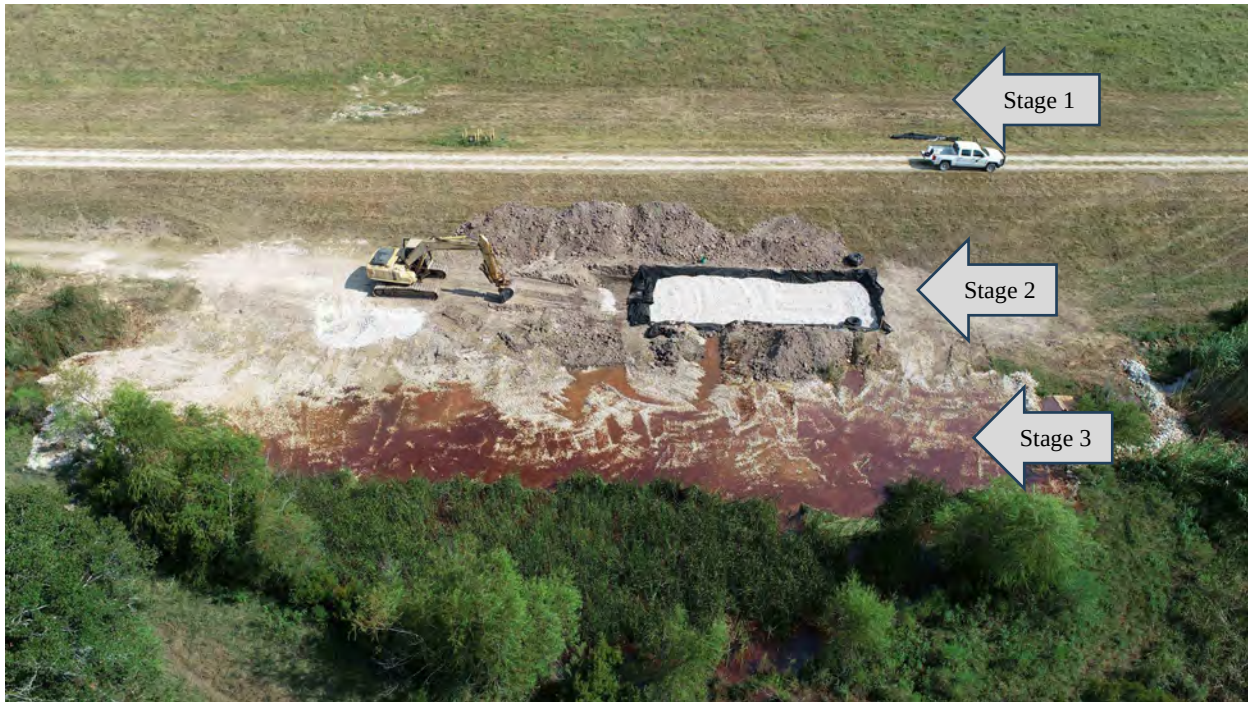
Figure 6 – Seep 1A Mitigation Progress (8/31/23)
