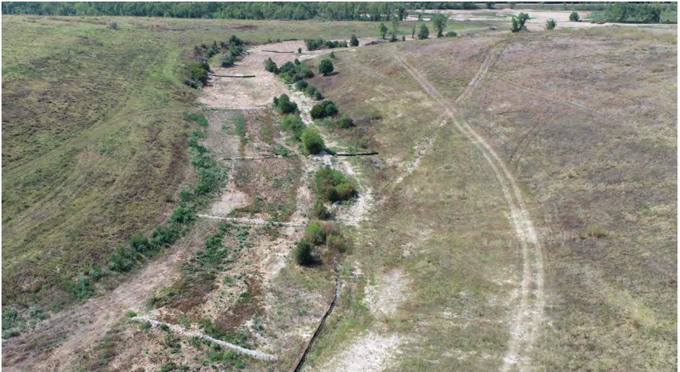
Figure 4 – Seep 9A area after mitigation (08/31/23)
