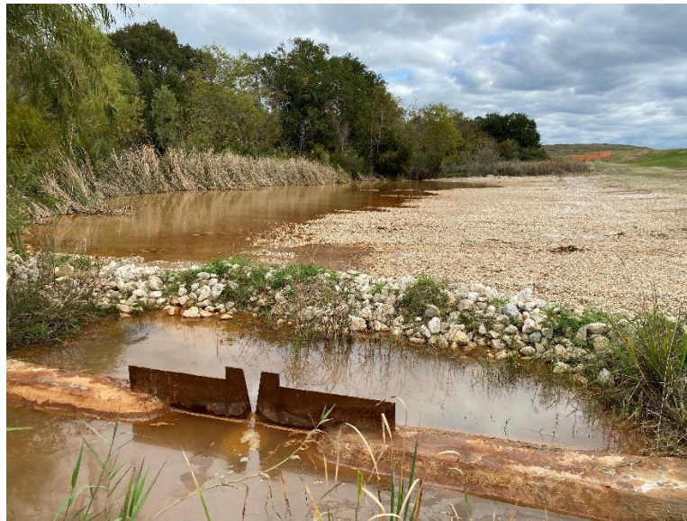
Figure 6 – Seep 1A gravel bed (right) and wetland (left) after reclamation. V-notch weir in foreground (view northeast, 11/21/23)
