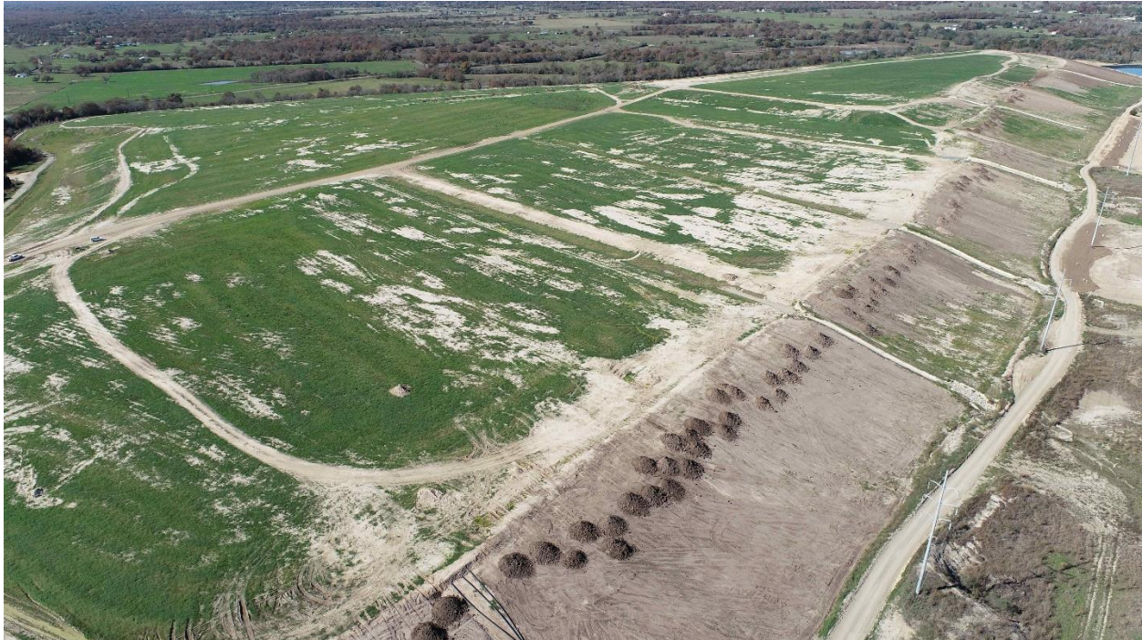
Photo 1: Site A Landfill – Vegetation becoming established on top and repairs to side slopes in progress (December 2023)
