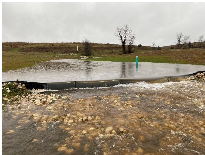
Figure 3 – Lowermost berm with greatest flow in Seep 9A drainage (Green stand-pipe marks location of original V-notch weir monitoring station; view south, 01/24/24 at 9:45 AM)
