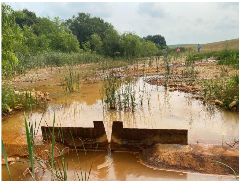
Figure 7 – Seep 1A – V-notch weir at discharge (view northeast, 05/28/24)
