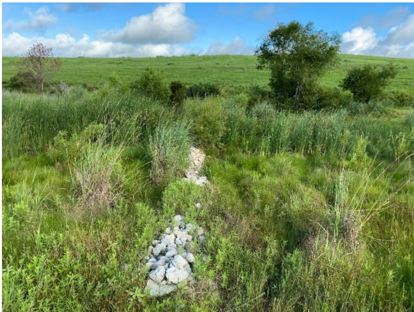
Figure 2 – Limestone berm to stabilize soil and reduce erosion (view west, 06/25/24)
