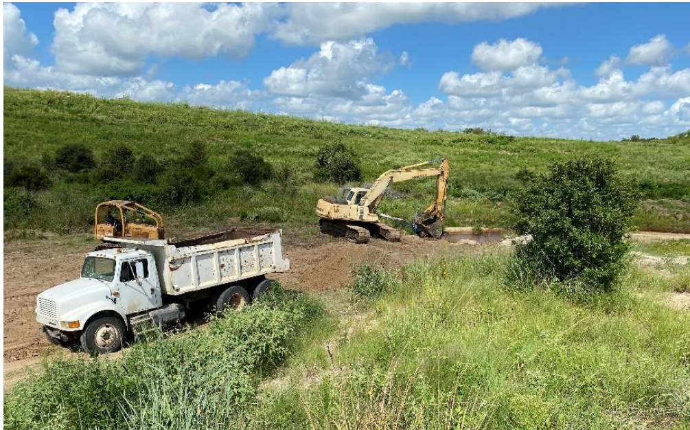
Figure 4 – Erosion repair work at the lower end of the Seep 9A drainage (View northwest, 08/14/24)
