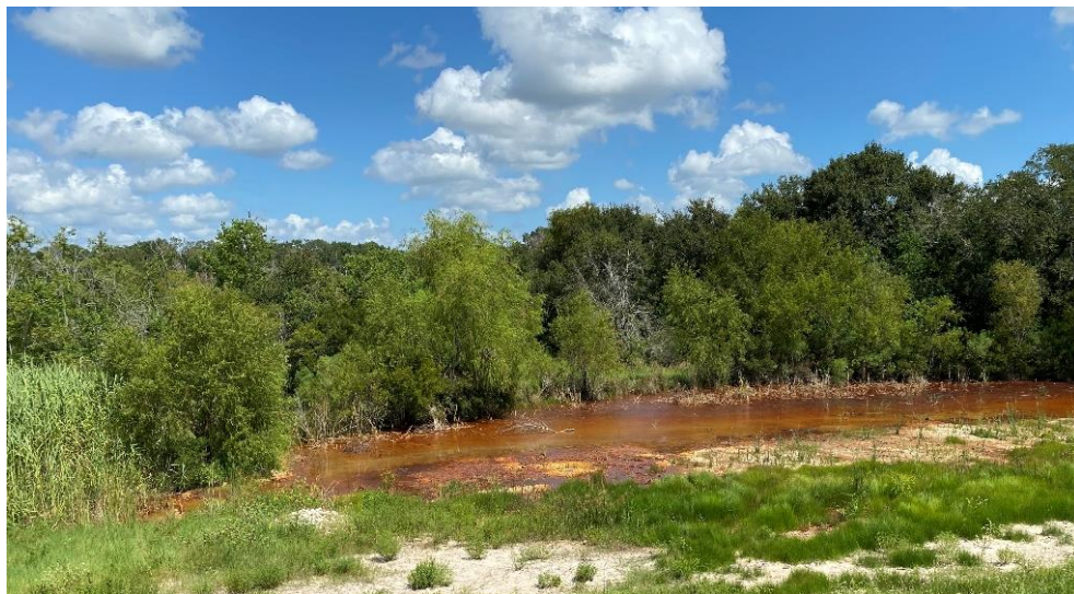
Figure 6 – Seep 1A – General view of wetland treatment area (view northeast, 08/14/24)
