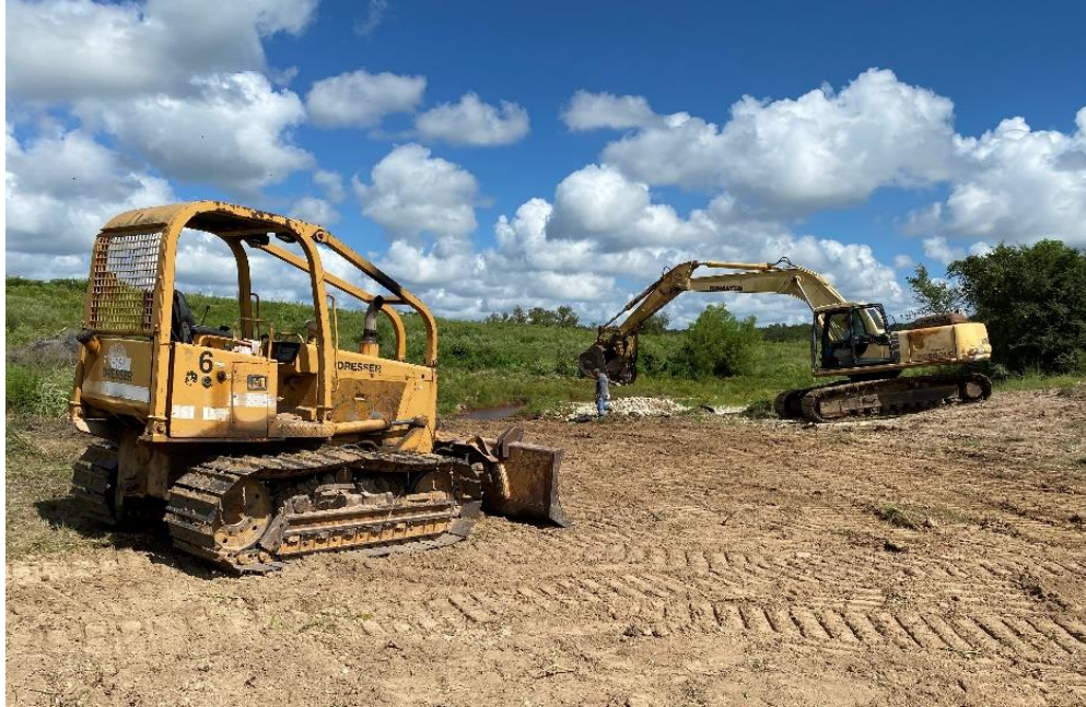
Figure 3 – Erosion repair work at the lower end of the Seep 9A drainage (View north, 08/14/24)
