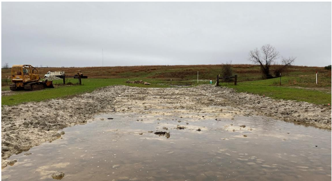
Figure 1 – Erosion control structure with grouted riprap at bottom end of Seep 9A drainage, constructed in October 2024 (View south, 02/12/25)
