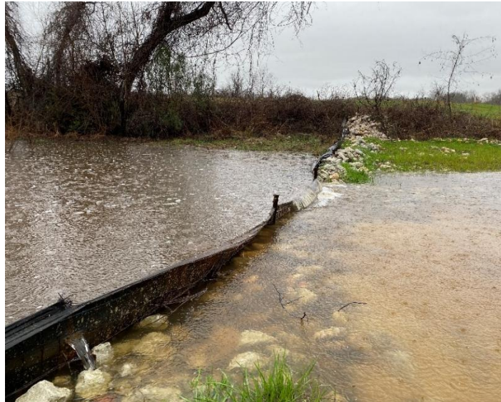
Figure 2 – Performance of silt fence and grouted riprap apron near bottom end of Seep 9A drainage during rain event (View west, 02/12/25)
