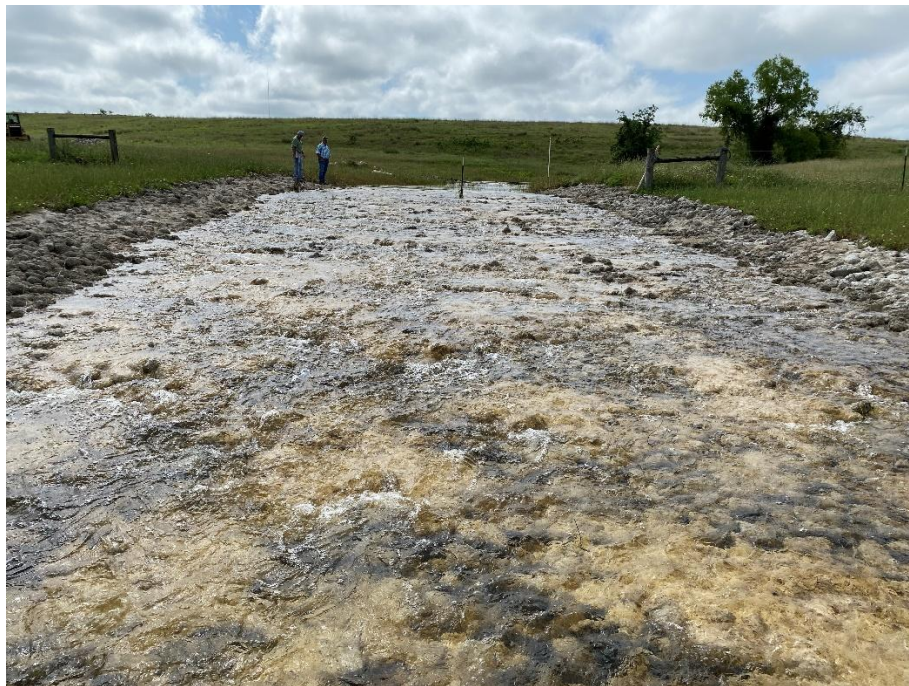
Figure 3 – Grouted riprap erosion control structure at bottom end of Seep 9A drainage (View south, 05/7/25)
