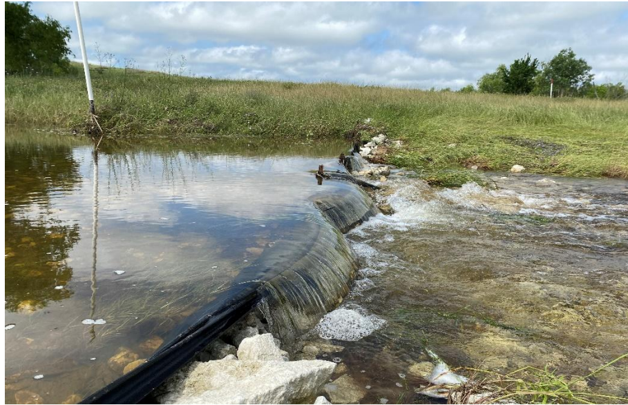
Figure 2 – Silt fence in Seep 9A drainage after large rain event (View west, 05/7/25)
