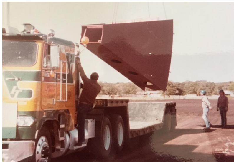
Delivery of first parts for the dragline, November 10, 1980
