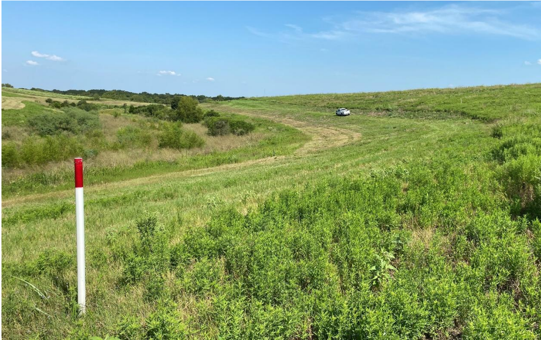
Figure 2 – Vegetation in the bottom of the Seep 9A drainage (Red-topped pipe marks the boundary between the area still bonded to the left, and the area released from bonding to the right) (View north, 08/25/25)
