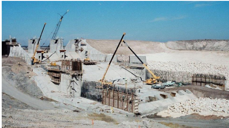
Construction of the Principal Spillway, Gibbons Creek Reservoir, Summer 1980
