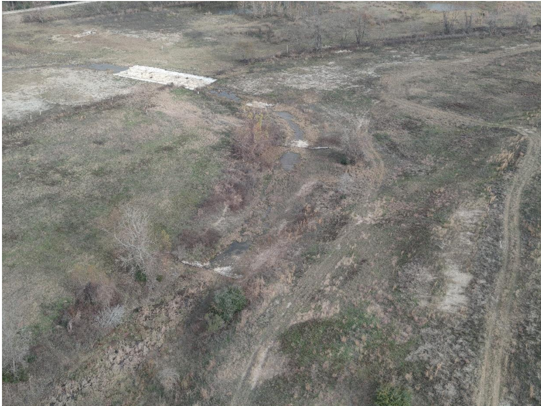
Figure 4 – Vegetation in lower section of Seep 9A mitigated in 2023 (grouted riprap erosion control structure visible at downstream end) (View northeast, 01/6/26)
