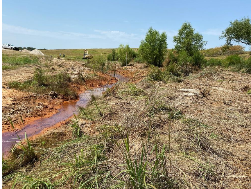
Figure 4 – Seep 9A just before start of mitigation (View south looking upstream, 07/18/22)
