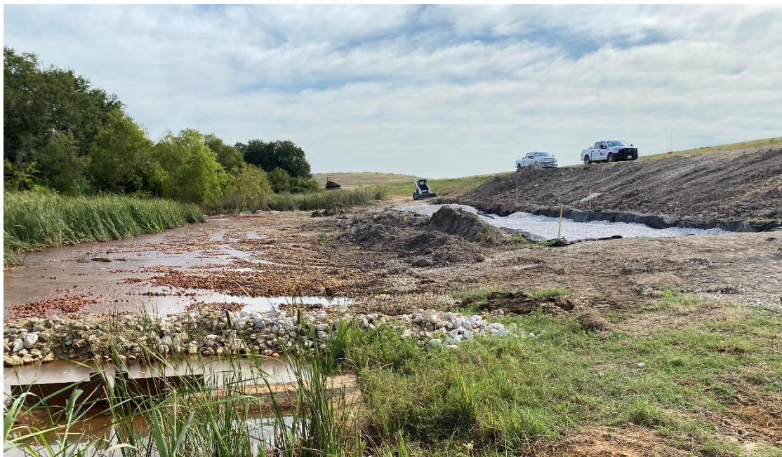
Figure 1 – Seep 1A mitigation in progress, wetland area to the left (View northeast, 09/11/23)
